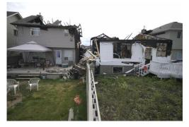
Building separations are addressed in the building codes under limiting distances. The code does not have a defined separation distance but instead talks about what is permitted for percentage openings based on what the limiting distances is.
