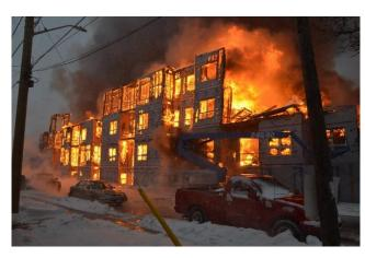
Homes in our communities are most vulnerable when they are under construction. Buildings do not have their complete fire safety systems in place such as compartmentalization, fired rated assemblies, and fire safety systems. Complicating the matter, calculated required fire flows do not consider this increased demand. Communities are
