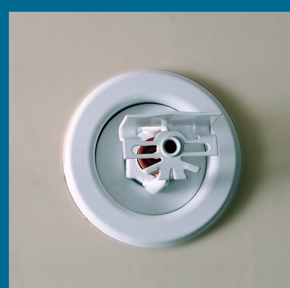
Sidewall Sprinkler
